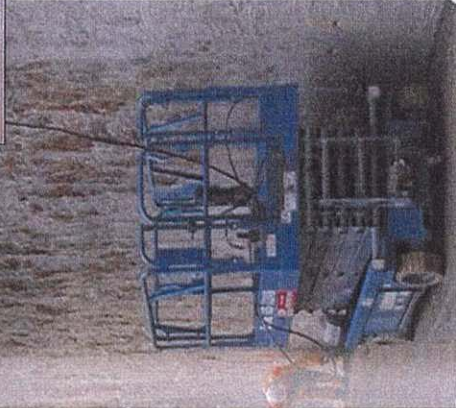
Exposed diaphragm walls can often form the final internal finish of underground structures.
