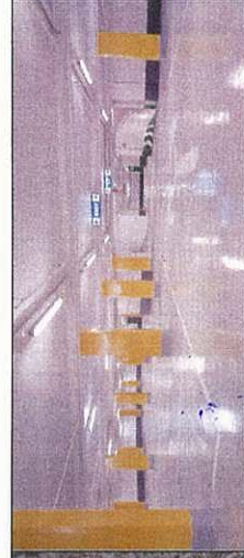
Exposed diaphragm walls can often form the final internal finish of underground structures.
