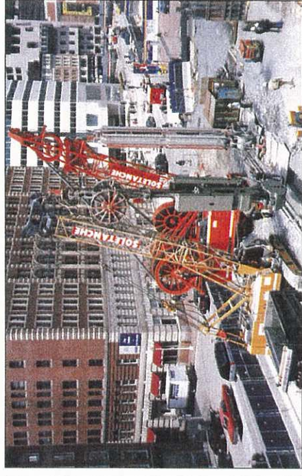
Hydrofraise diaphragm wall construction can be fast, even in difficult ground.
