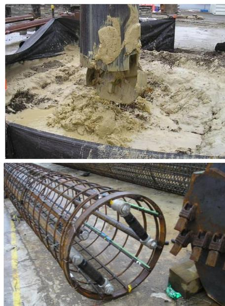
Figure 2b: Pile spoil grouting pipe work
