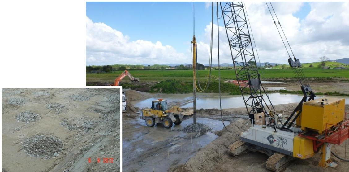
**Figure 5: Vibroreplacement installation**
